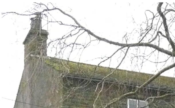
**Figure 57 Stone Slate Roof With Stone Chimney and Clay Pots**
