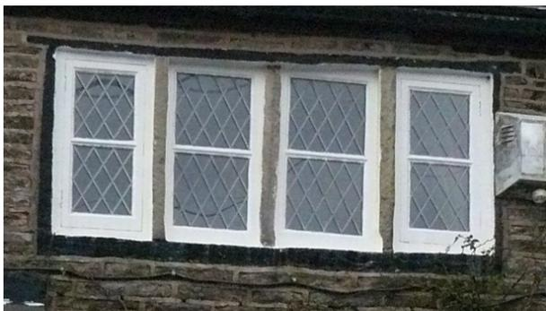
**Figure 46 Side-opening Casement Window**
