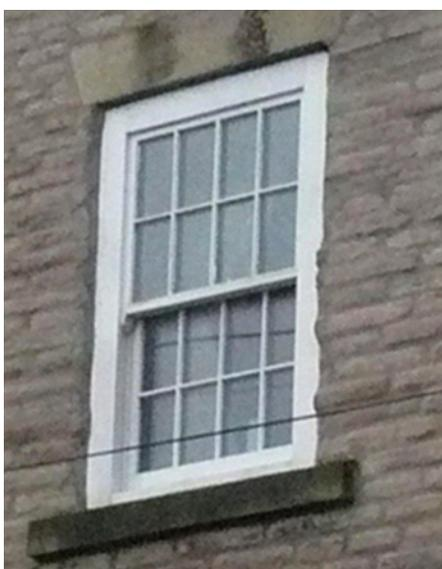
**Figure 47 Eight-Over-Eight Sash Window, After c1850**
