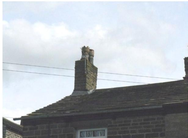
**Figure 61 Stone Slate Roof With Stone Chimney and Clay Pots**
