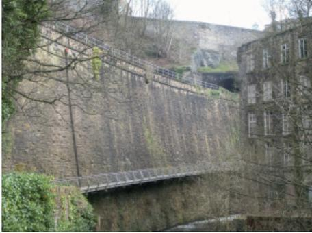
**Picture 22** Vast retaining wall supporting the Manchester-Sheffield railway
