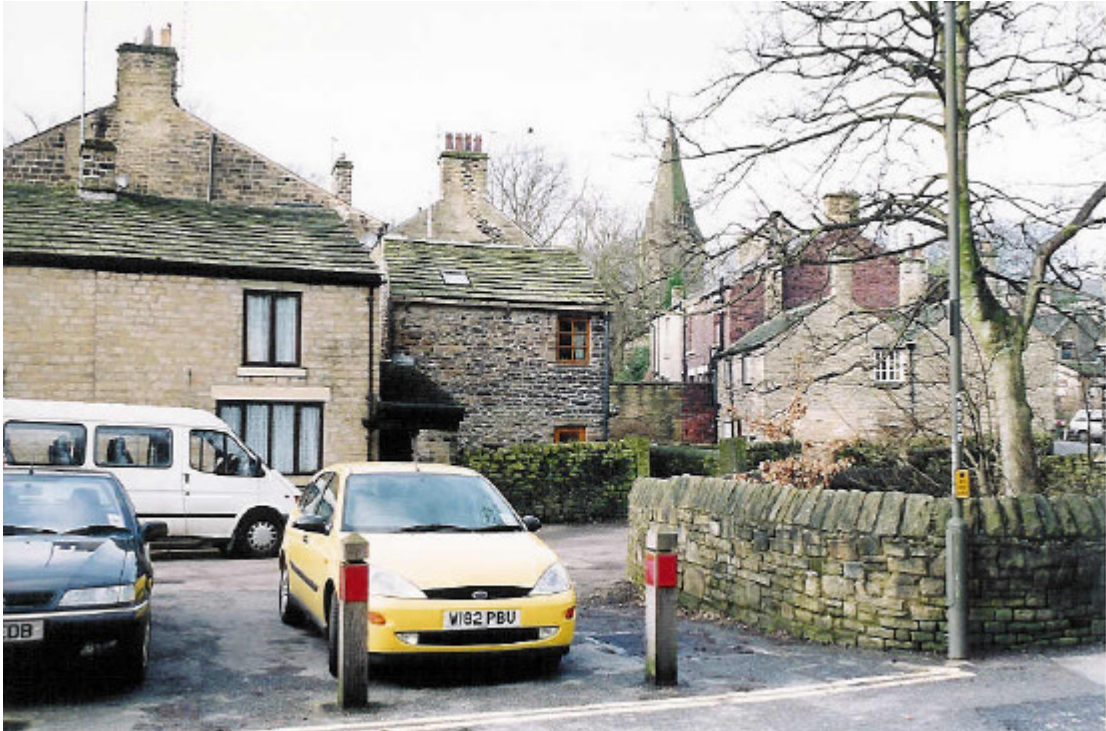
Stone Slate Roofs in historic core
