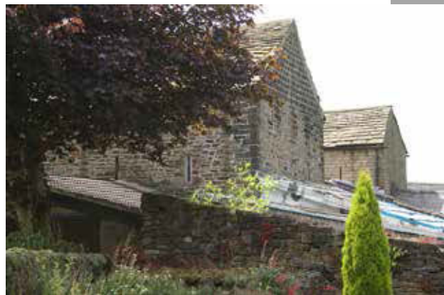
Two phases of barns behind Padfield Main Road. The barn in the foreground is 17th century in origin and retains the characteristic ,stacked, narrow ventilation slits and irregular quoins.
