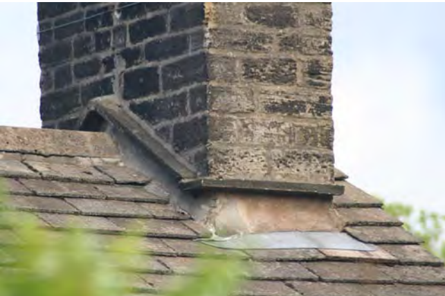
“Water tabling” to the stone chimneys (left) & moulded timber “trow” on timber eaves corbels (right)
