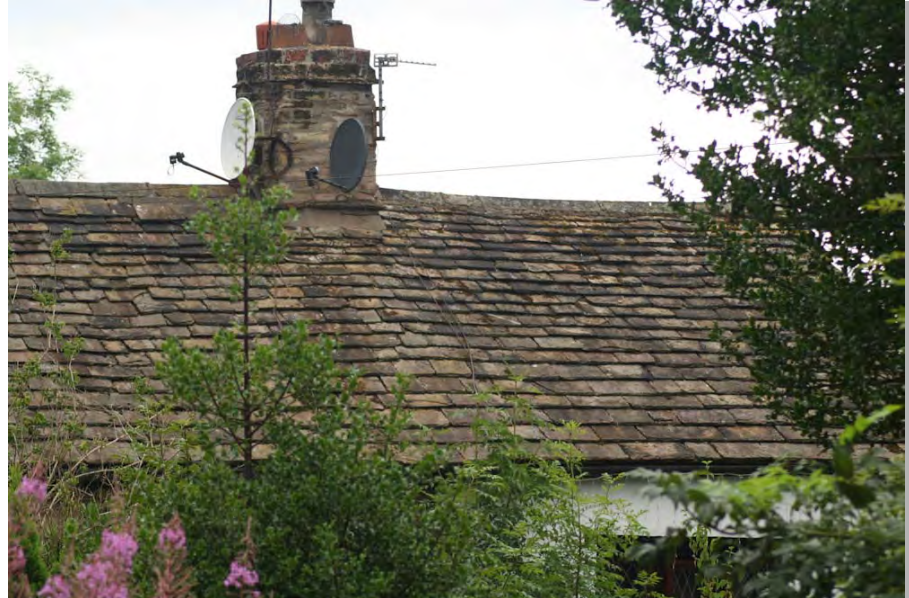
Local graduated stone slate roofs
