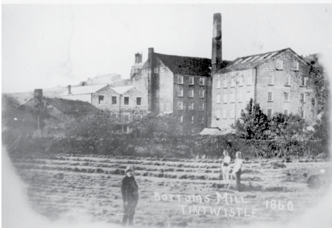
Bottoms Mill of c.1820, photographed before demolition in 1864 (courtesy Glossop Heritage Trust)
