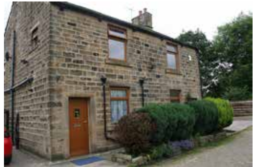
Arnfield House, Arnfield Lane (a former pair of cottages with watershot masonry)
