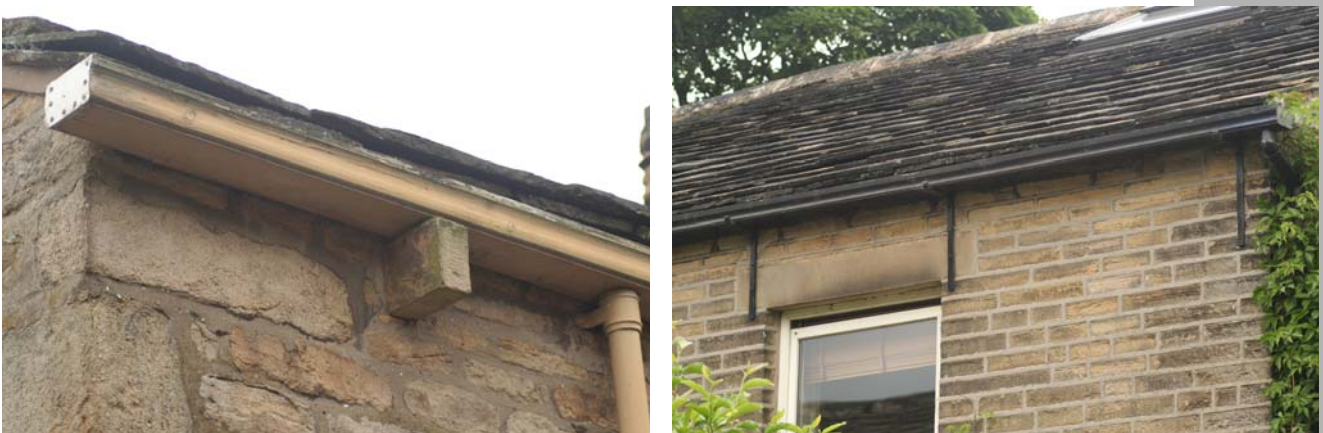
Timber gutters (“trows”) are traditionally fixed on stone corbels (left) or metal brackets (right)
