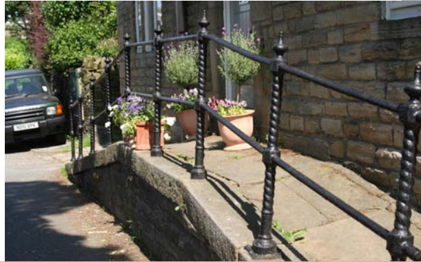
Cast-iron stanchions combined with iron rails (above) and wrought iron gates (below)
