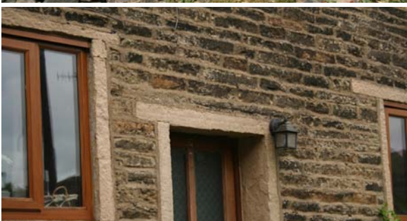
The local fissile stone is used for drystone boundary walls, graduated stone slate roofs & stone dressings
