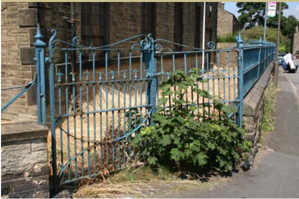
Cast-iron stanchions combined with iron rails (above) and wrought iron gates (below)
