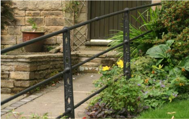
Cast-iron stanchions combined with iron rails (above) and wrought iron gates (below)
