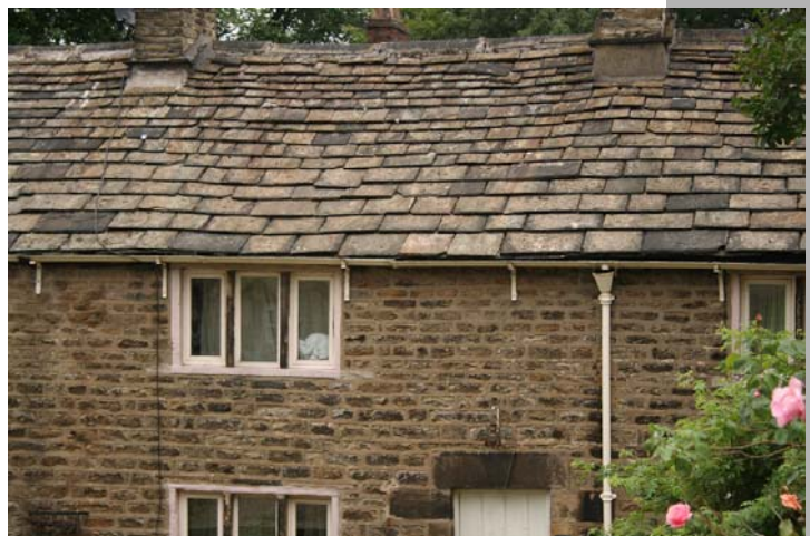
The local fissile stone is used for drystone boundary walls, graduated stone slate roofs & stone dressings
