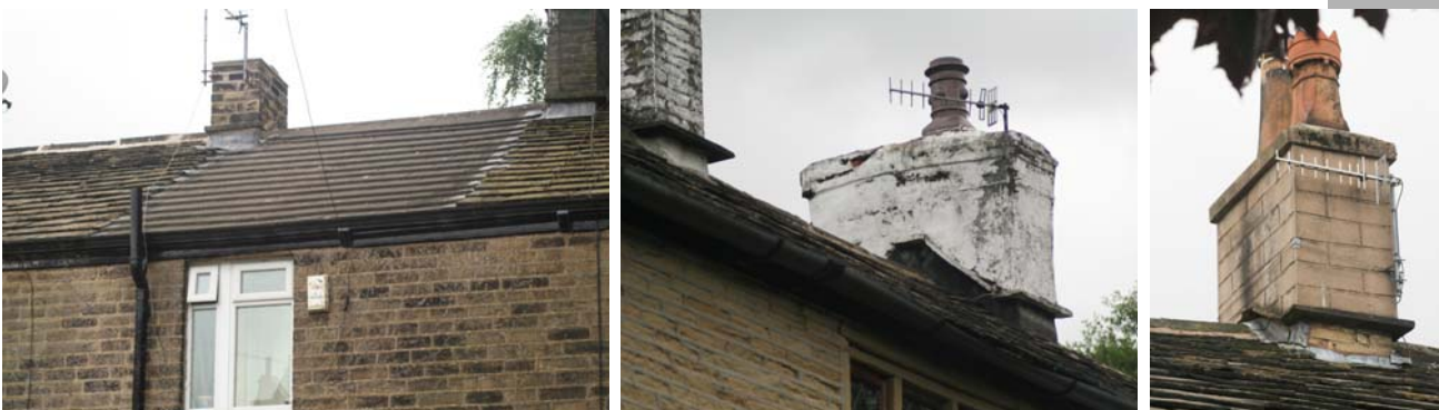
From left - artificial stone (concrete tiles) and rendered stacks covering original stonework
