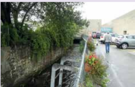
River Wye in hidden culvert
