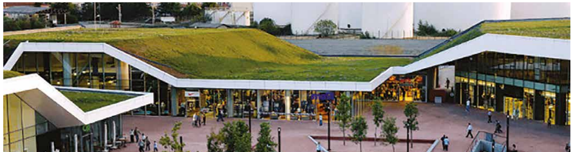
Green roofs and podium gardens
