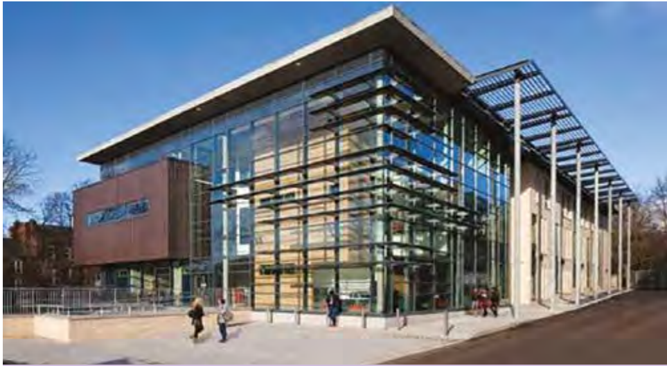
New College Building
