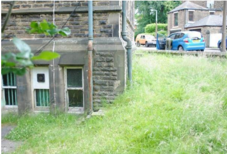
FIGURE 17 – PHOTOGRAPH ILLUSTRATING HOW THE EXTERNAL LOWER GROUND FLOOR WALL WHICH IS ACTING AS A RETAINING WALL. THE INTERNAL FACE OF THIS WALL IS DAMP.
