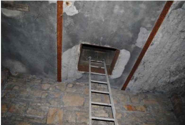
FIGURE 52 – EXAMPLE OF CORROSION TO STEELWORK
