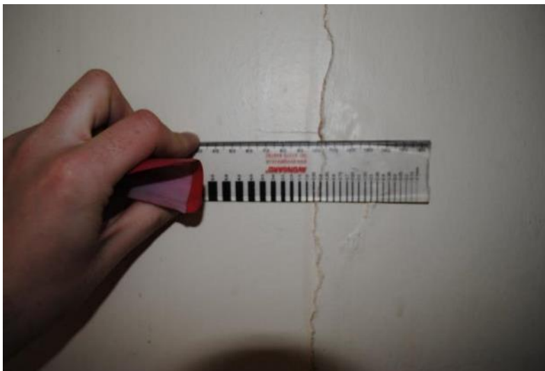
FIGURE 45 – CRACKING IN PLASTER, THOUGHT TO BE ATTRIBUTABLE TO WATER INGRESS
