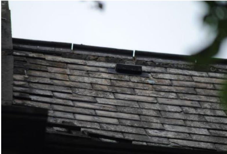
FIGURE 21 –EXAMPLE OF DAMAGED ROOF TILES, SOME HAVE SLIPPED OUT OF PLACE.
