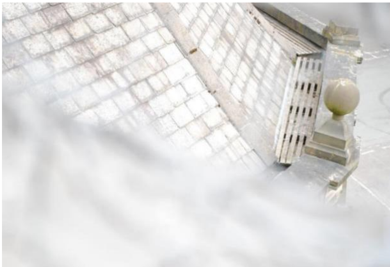
FIGURE 55 – VIEW OF PARAPET GUTTER FROM THE TOWER
