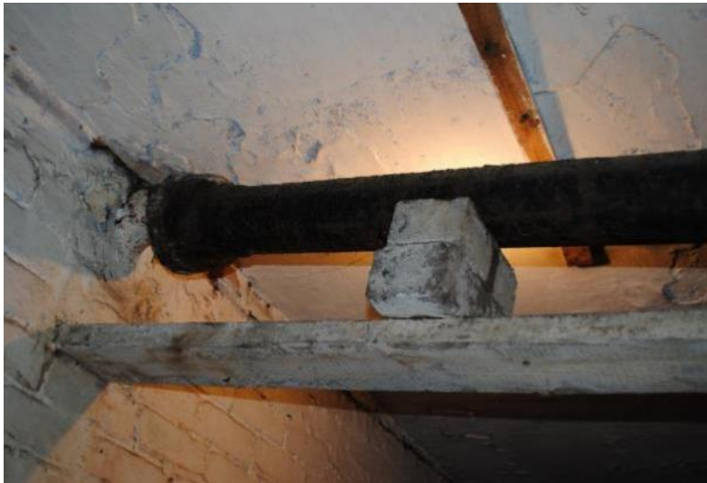
FIGURE 31 – POORLY DETAILED PIPE SUPPORT STRUCTURE REQUIRES ADDRESSING
