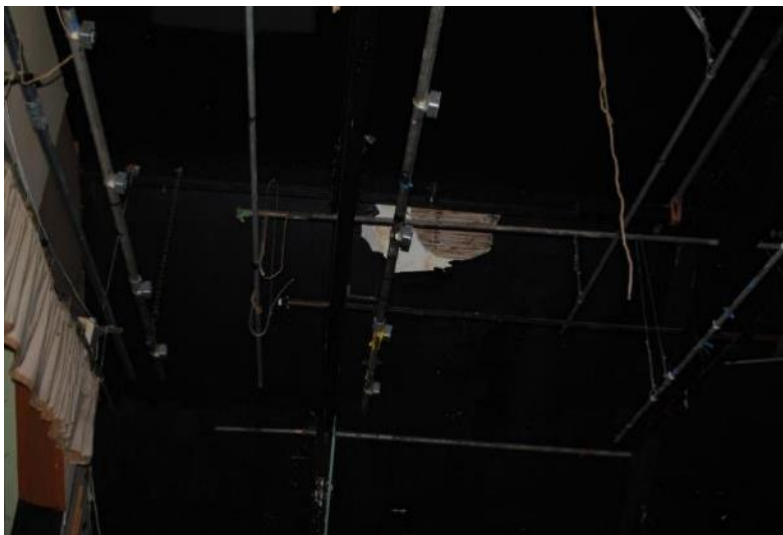
FIGURE 47 – PARTIALLY COLLAPSED CEILING ABOVE THE STAGE
