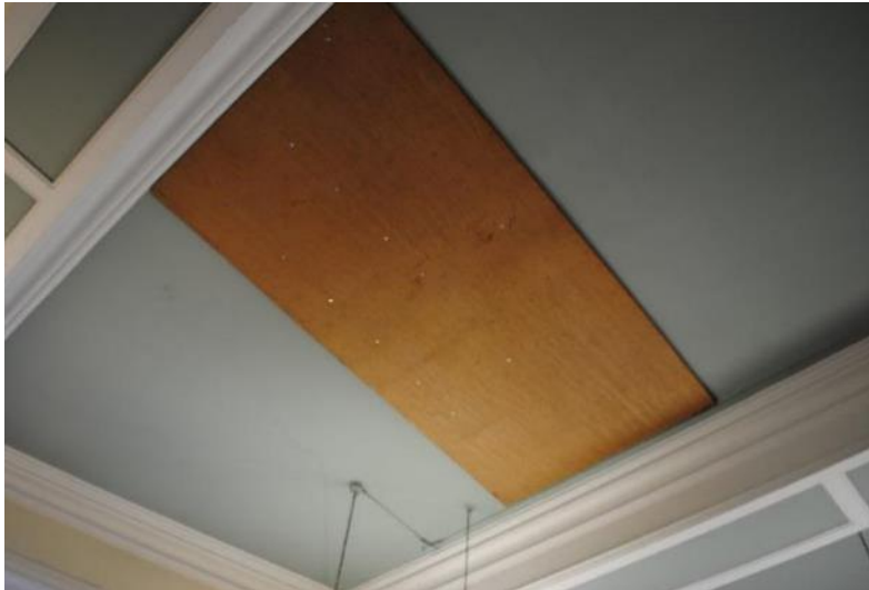
FIGURE 35 – EXAMPLE OF PLYWOOD BOARD ATTACHED TO CEILING TO PROVIDE A TEMPORARY REPAIR
