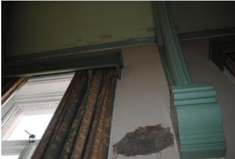
FIGURE 46 - EXAMPLE OF WATER DAMAGE TO PLASTER
