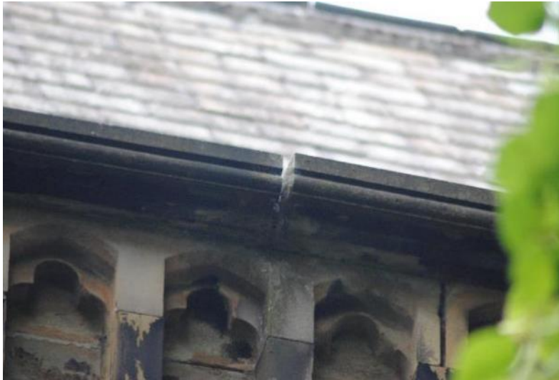
FIGURE 23 – EXAMPLE OF MOVEMENT AND CRACKING IN PARAPET WALL.
