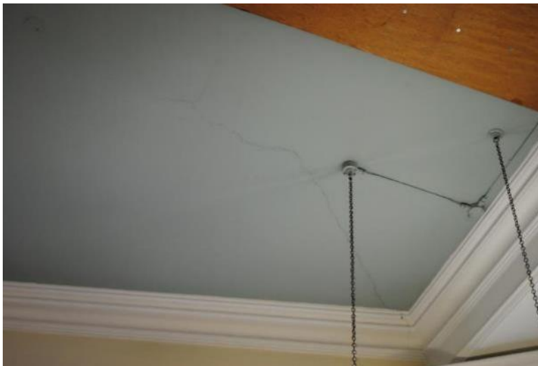
FIGURE 36 – EXAMPLE OF HAIRLINE CRACKING IN THE CEILING FINISHES
