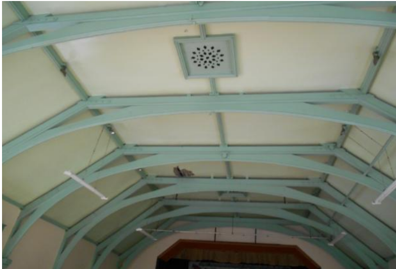
FIGURE 42 - ROOF OF FIRST FLOOR HALL
