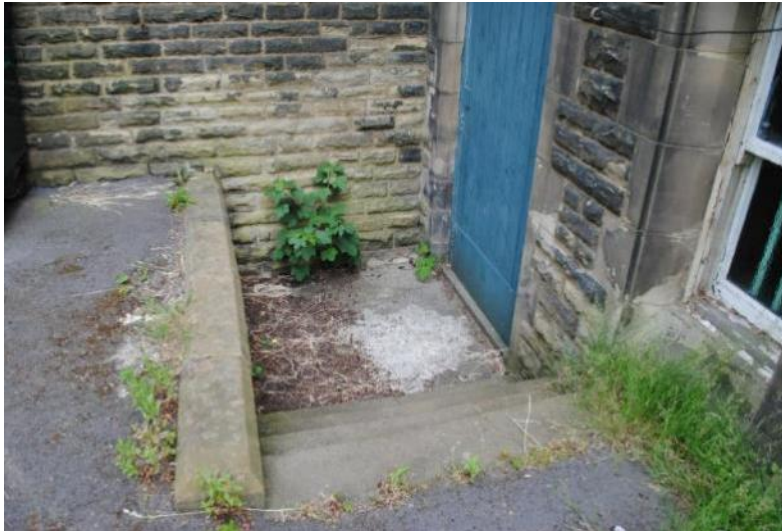
FIGURE 15 – EXAMPLE OF ACCESS TO THE LOWER GROUND FLOOR. THE SURFACE WATER GULLEY IS BLOCKED, VEGETATION IS GROWING IN THE GULLEY AND THE DOOR THRESHOLD HAS FAILED.
