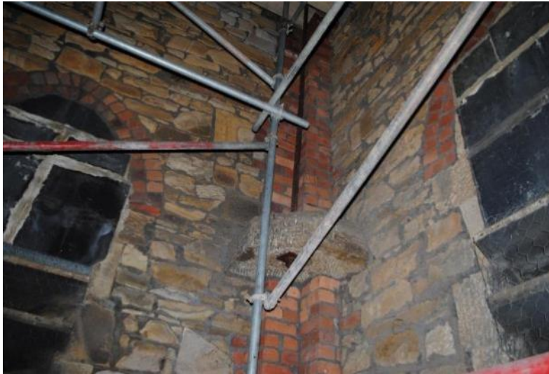
FIGURE 54 - TOWER STRUCTURE IS SECURED BY FOUR CAST IRON TIE BEAMS, HELD BY CONCRETE SUPPORTS.
