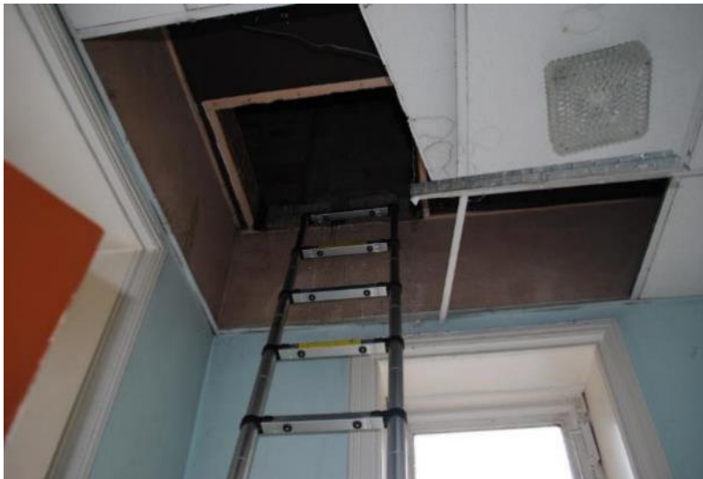
FIGURE 49 – ACCESS TO THE TOWER
