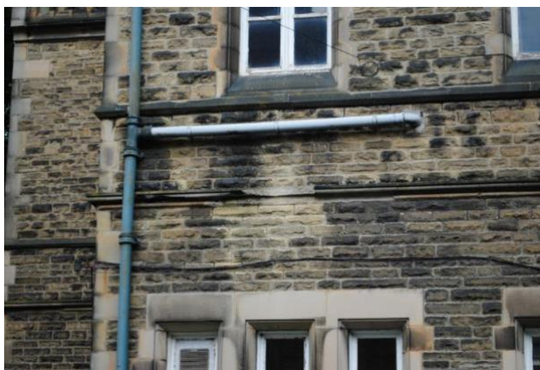
FIGURE 9 – EXAMPLE OF BROKEN BAND COURSE
