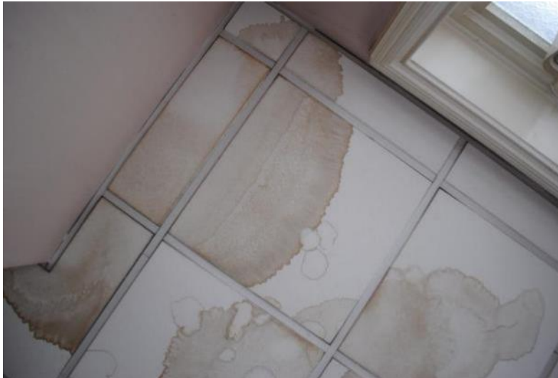
FIGURE 50 - WATER DAMAGE TO CEILING OF WOMEN'S BATHROOM.
