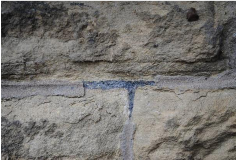
FIGURE 6 – TYPICAL EXAMPLE OF THE POINTING TO THE FACING STONework. EARLIER LIME/ASH MORTAR IS EVIDENT BEHIND THE MOST RECENT REPOINTING.
