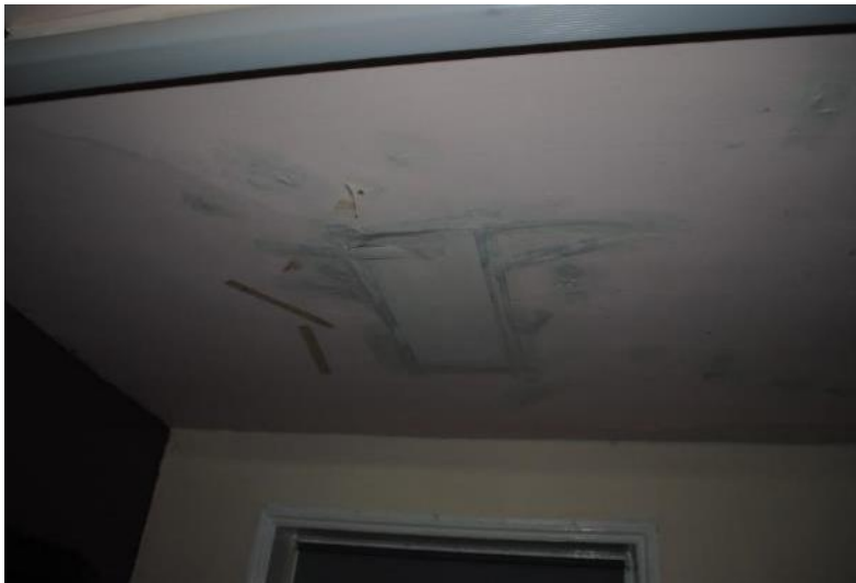
FIGURE 28 – EXAMPLE OF PREVIOUS POOR QUALITY REPAIRS TO CEILINGS
