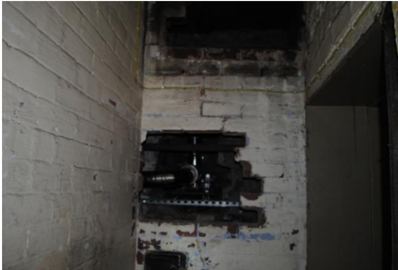
FIGURE 25 – MECHANICAL SYSTEMS BUILDER’S WORK HAVE BEEN POORLY COMPLETED. A LINTEL IS REQUIRED TO THIS PIPE OPENING.
