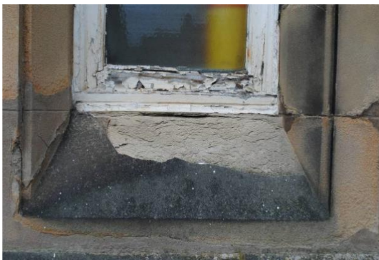
FIGURE 5 –TYPICAL EXAMPLE OF THE CONDITION OF WINDOW FRAMES
