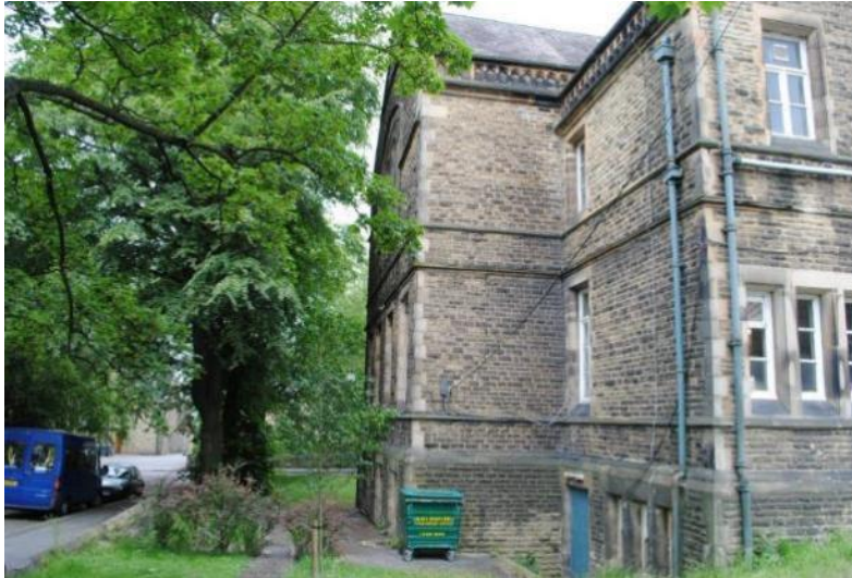
FIGURE 4 –SOUTH ELEVATION ILLUSTRATING THE PROXIMITY OF TRESS IN THE SOUTH-WEST CORNER
