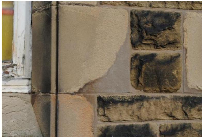
FIGURE 8 - EVIDENCE OF PREVIOUS REPAIRS OF THE STONE BLOCKS.
