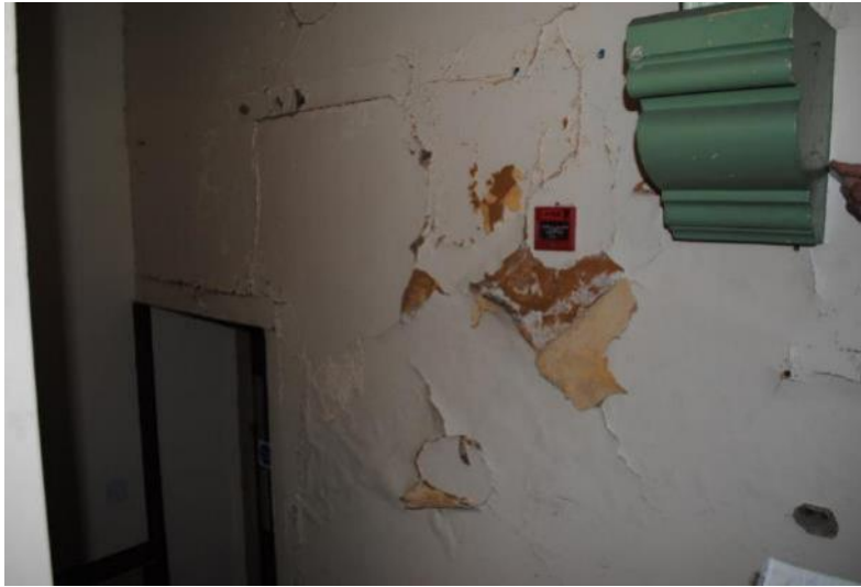
FIGURE 48 – EXAMPLE OF WATER DAMAGE
