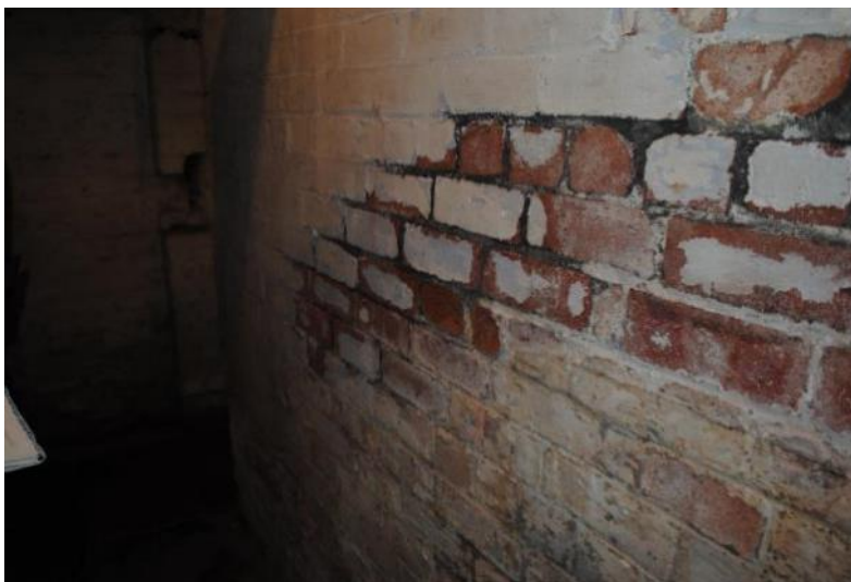
FIGURE 32 – EXAMPLE OF SOFT BRICKS IN DAMP WALL
