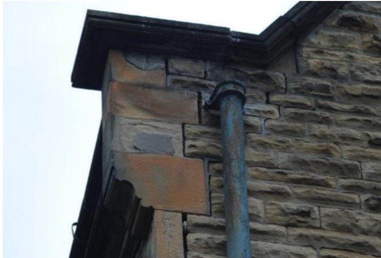
FIGURE 10 – EXAMPLE OF LOOSE POINTING, OPEN JOINTS AND MOVEMENT IN STONework AT PARAPET LEVEL. THIS DEFECT OCCURS IN MULTIPLE LOCATIONS.
