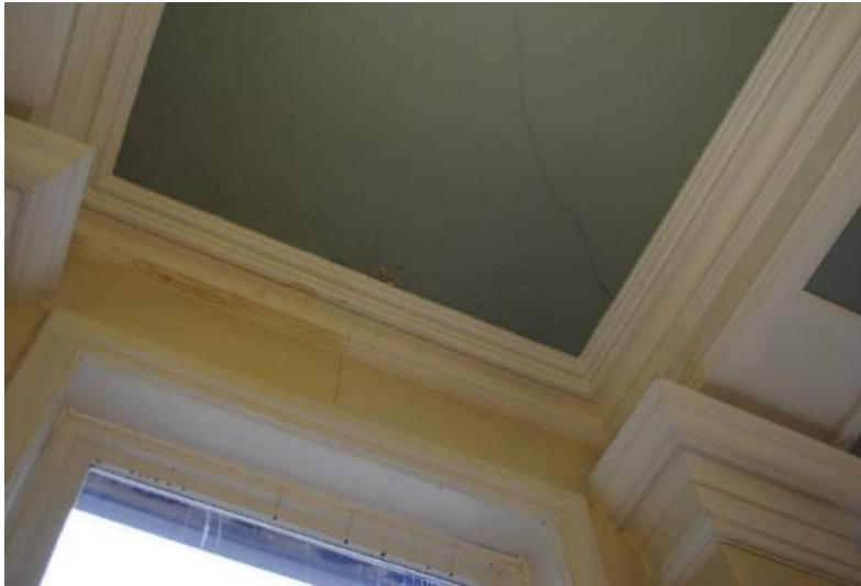
FIGURE 37 – EXAMPLE OF WATER INGRESS
