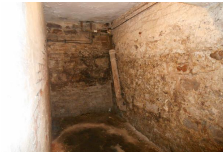
FIGURE 30 - FURTHER EVIDENCE OF DAMP. FLOOR HAS AN ASPHALT COVERING, WHICH SUGGESTS PAST INEFFECTIVE ATTEMPTS TO ADDRESS DAMP ISSUES.
