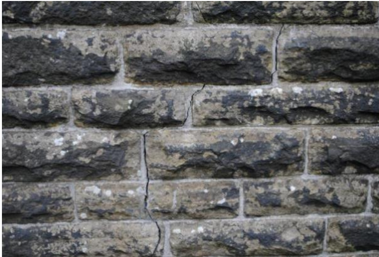
FIGURE 13 – EXAMPLE OF MINOR SETTLEMENT CRACKING
