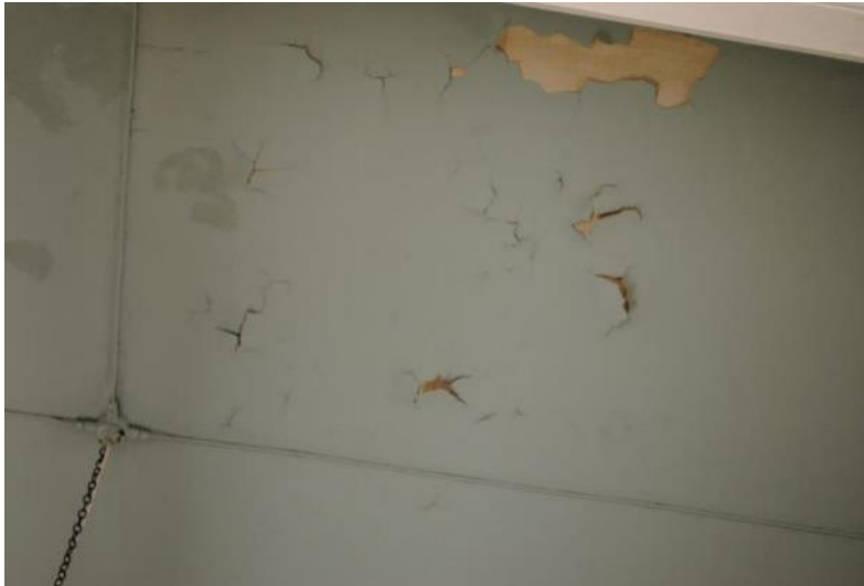
FIGURE 39 – EXAMPLE OF WATER DAMAGE TO CEILING.
