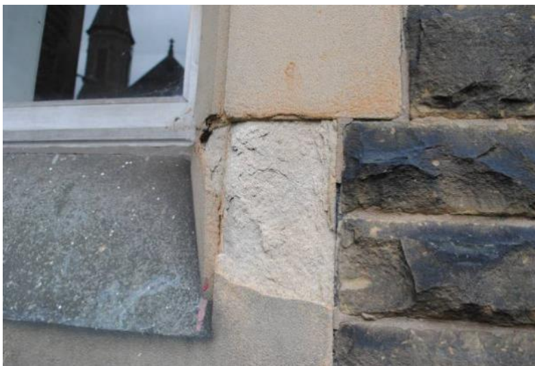
FIGURE 7 – TYPICAL EXAMPLE OF STONework WITH A SPALLED FACE
