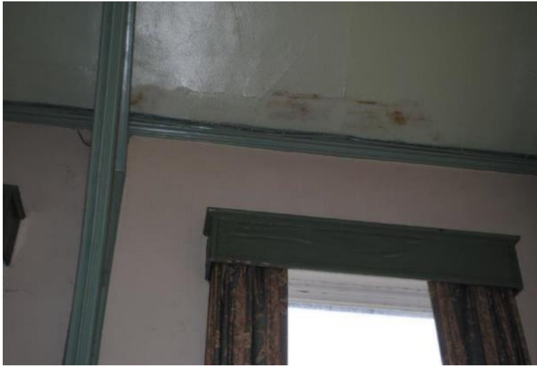
FIGURE 44 – EXAMPLE OF STAINING. THE STAINING IS AT THE SAME LEVEL AS THE PARAPET GUTTER
