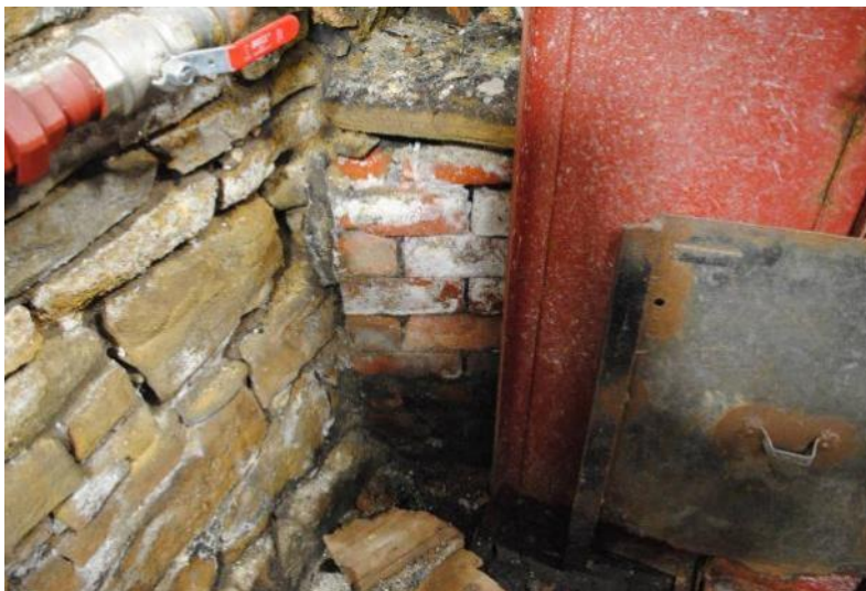
FIGURE 24 – EXAMPLE OF WATER INGRESS IN THE SHOWN BY DAMP BRICKWORK AND SALT STAINING
