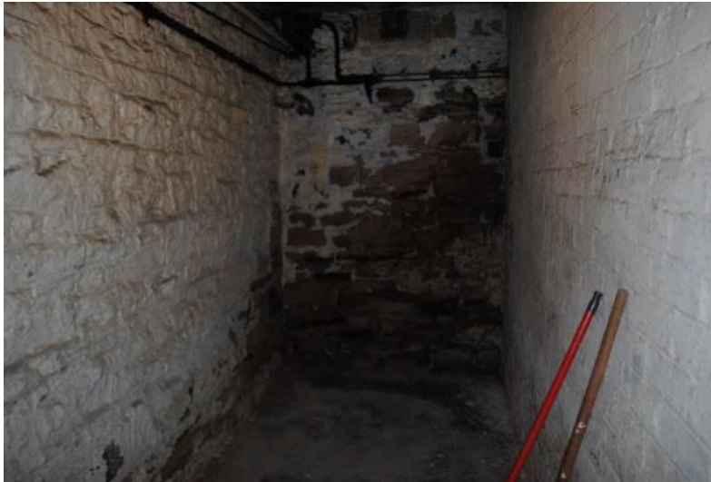
FIGURE 29 – EXAMPLE OF DAMP WALLS
