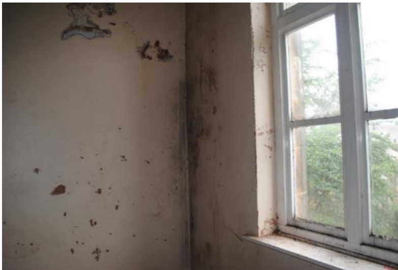
FIGURE 51 - FURTHER WATER DAMAGE TO WALLS
