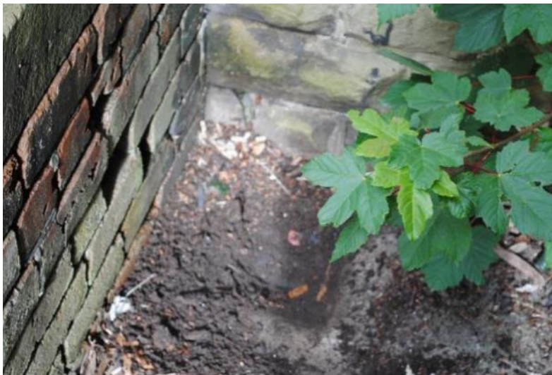
FIGURE 16 – EXAMPLE OF SILTED UP GULLEY
