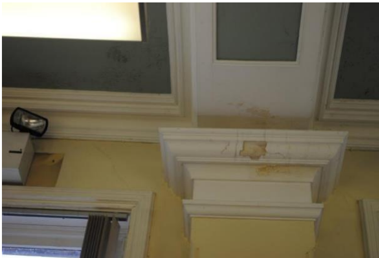
FIGURE 38 – EXAMPLE OF WATER INGRESS
