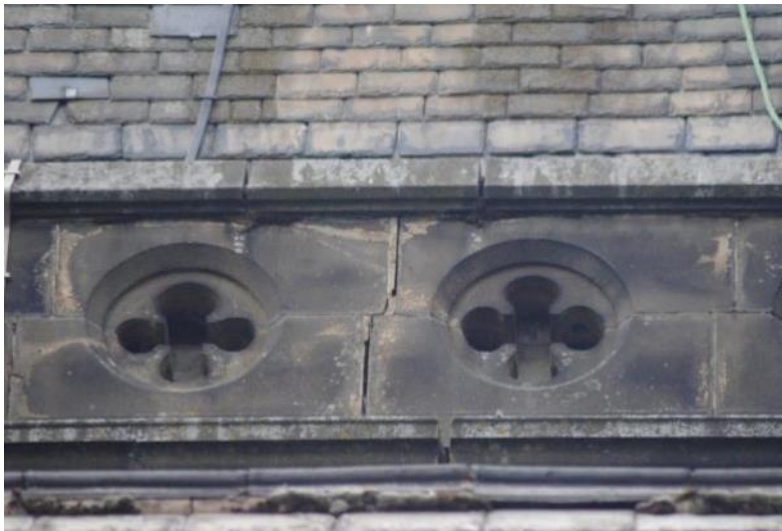
FIGURE 12 – EXAMPLE OF OPEN JOINTS AND LOOSE MORTAR AT THE PARAPET LEVEL OF THE TOWER
