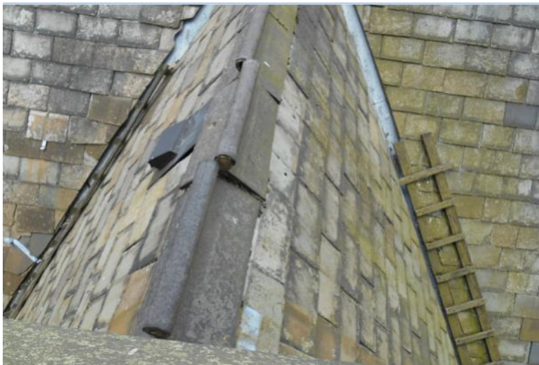
FIGURE 22 – EXAMPLE OF LOOSE RIDGE TILES
