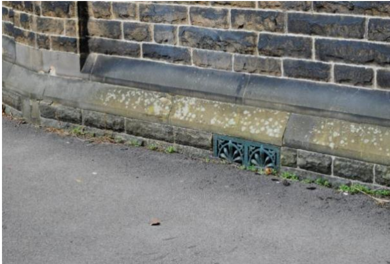
FIGURE 19 – EXAMPLE OF BLOCKED VENTILATION TO THE LOWER GROUND FLOOR
