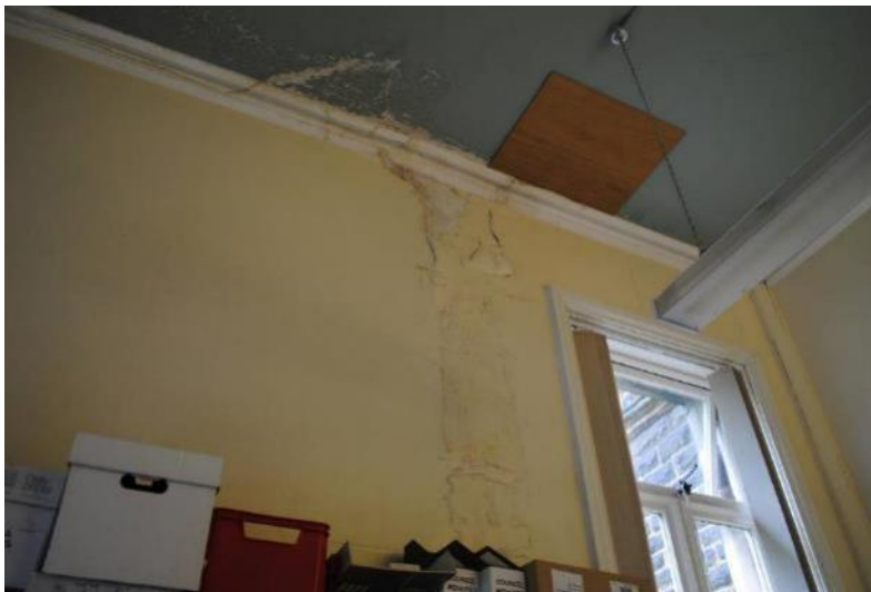
FIGURE 40 – EXAMPLE OF WATER INGRESS DAMAGE
