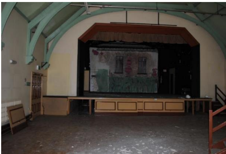
FIGURE 43 – ASSEMBLY HALL STAGE
