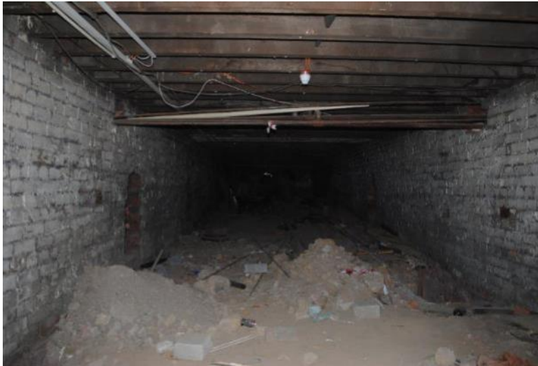
FIGURE 27 – SUB FLOOR VOID
