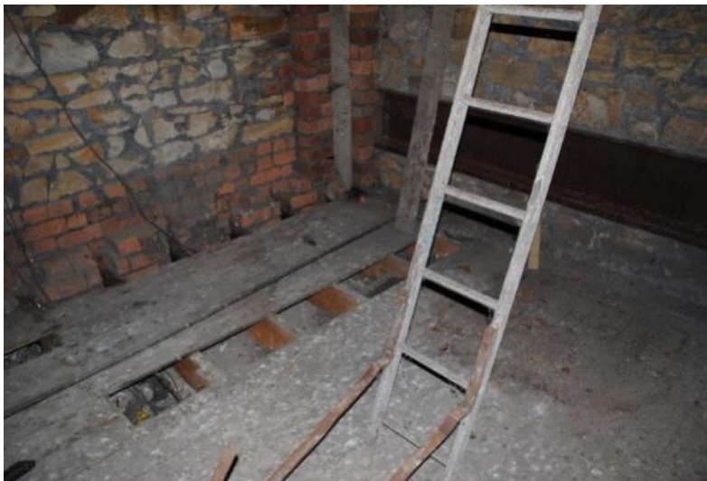
FIGURE 53 – TIMBER FLOOR COVERED IN PIGEON FOULING
