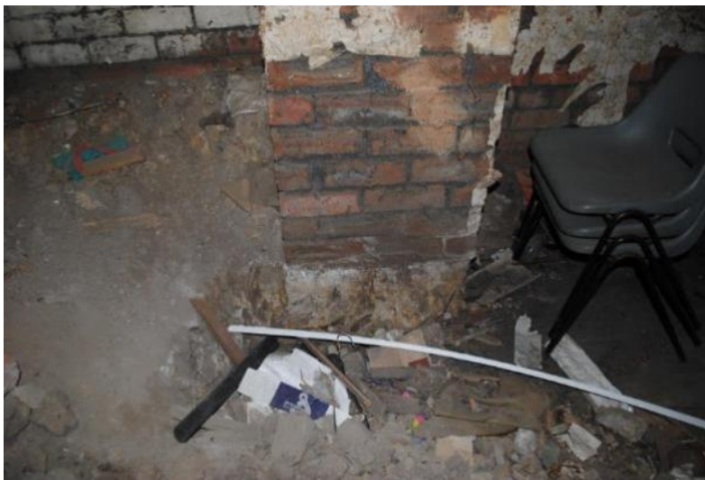
FIGURE 26 – EXAMPLE OF MASONRY BUILT DIRECTLY ONTO ROCK WITHIN THE SUB-FLOOR VOID.
