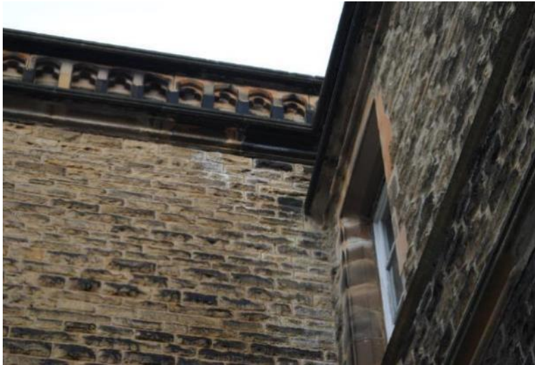
FIGURE 11 – EXAMPLE OF SALT STAINING IN THE STONework AT PARAPET LEVEL
