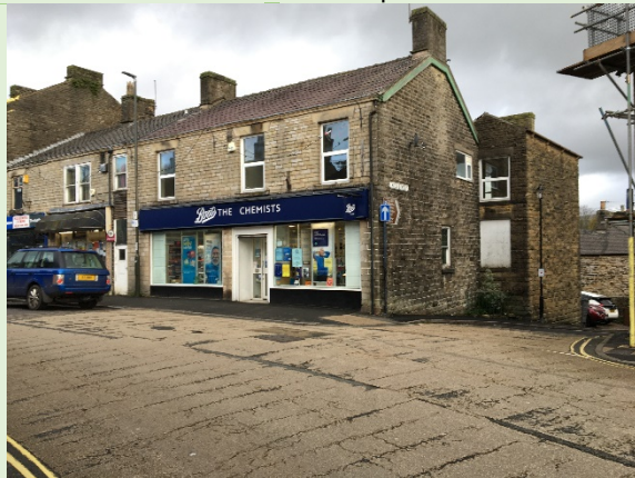
Figure 1: There are a number of attractive, well-maintained retail units in the town centre. These include both independent and national multiple operators, such as Boots on Market Street.
