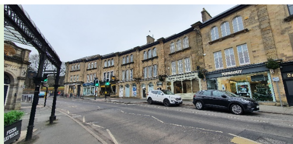
Figure 3: Crescent of retail units on Terrace Road
