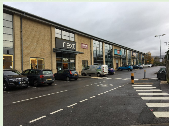
Figure 4: Wren Nest Retail Park, located in the west of the town centre, includes the converted former Wren Nest Mill which was redeveloped following a fire in 1996
