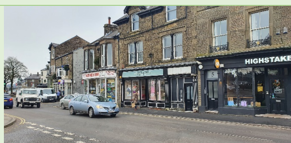
Figure 5: New Highstakes restaurant on High St
