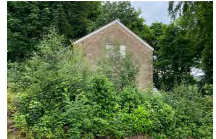
Photograph 8 - View of east elevation of the detached garage
