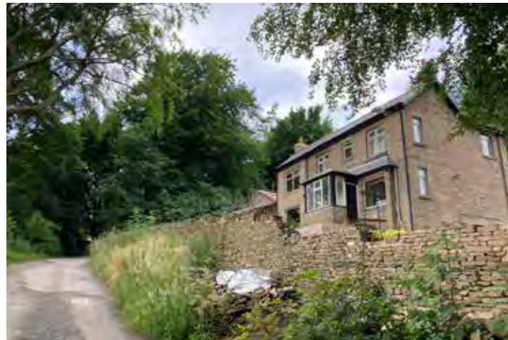
Photograph 5 - View of access driveway and Brewood
