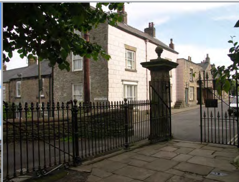
Former Bulls Head, Market Place, Chapel-en-le-Frith. The render has been incised so that it gives the appearance of ashlar stonework.
