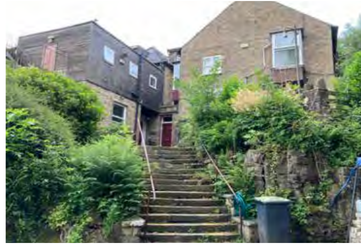
Photograph 10- View of east elevation of main house
