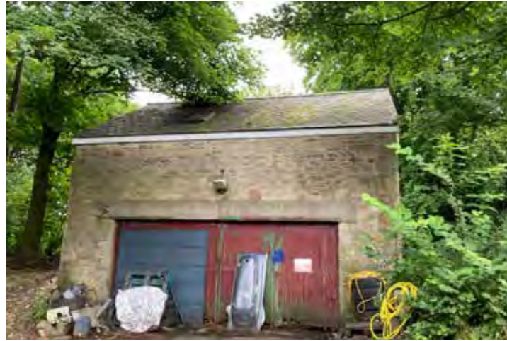
Photograph 9- View of south-west elevation of detached garage
