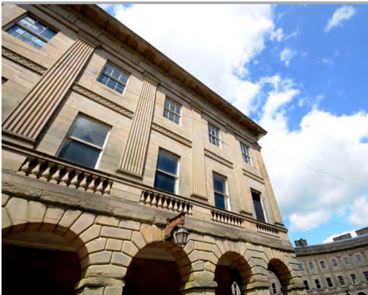
Crescent, Buxton, illustrating the use of ashlar gritstone in a variety of ways
