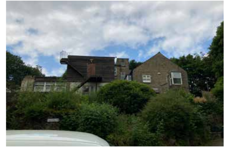
Photograph 12- View of east elevation of main house
