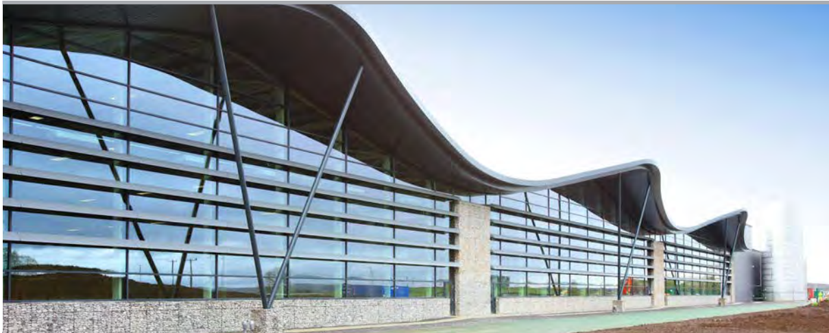
Buxton water bottling plant, Waterswallows, Buxton. A large building, well designed, using local natural materials to assimilate into the landscape.
