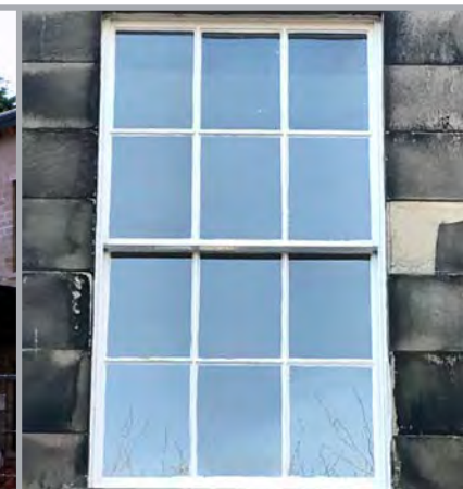
12 pane sash windows: each pane has the same vertical proportions as the window opening itself
