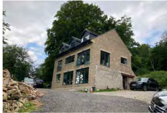
Photograph 14- Recent residential conversion (converted classroom - off site)
