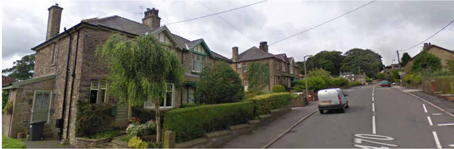
Photograph 16- Period semi-detached houses on Macclesfield Road
