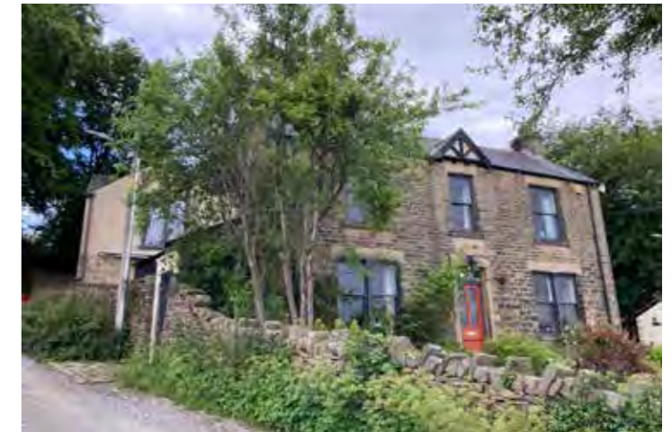
Photograph 4 - View of access driveway and front elevation of Woodside
