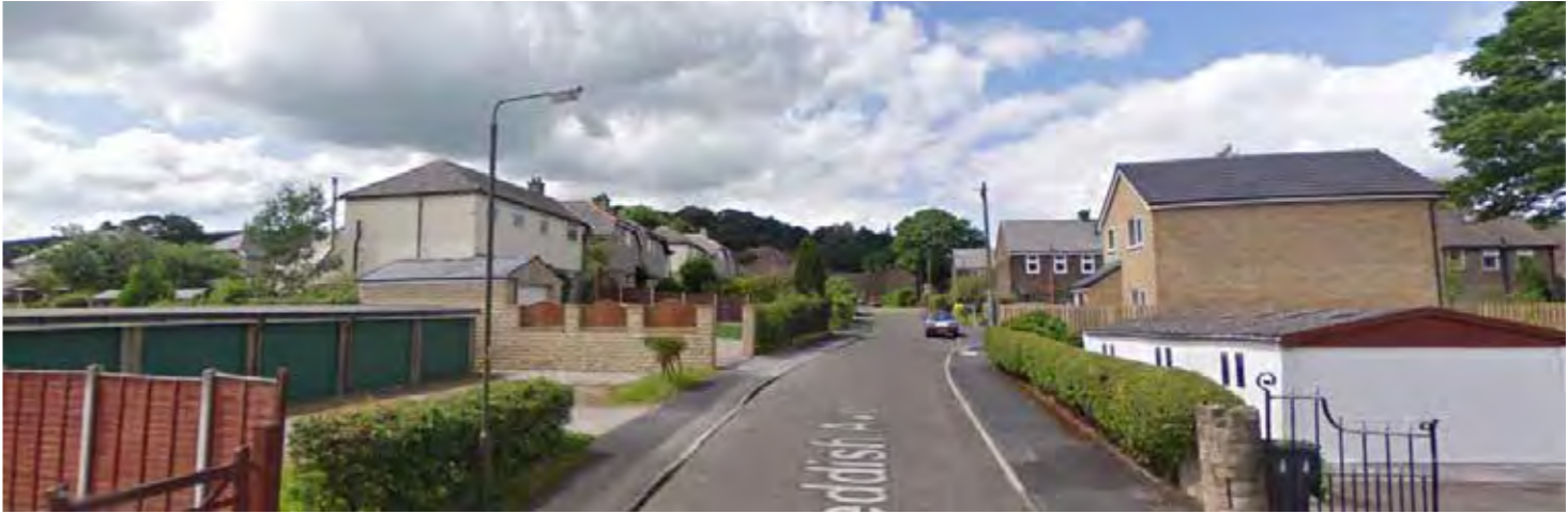
Photograph 19- Residential development on Reddish Avenue
