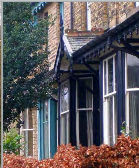
Sliding sash windows, Whaley Bridge.
