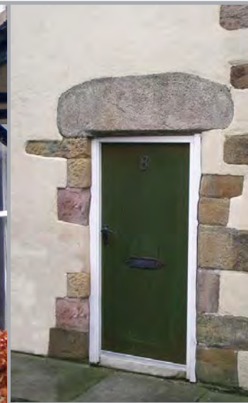
Early door opening (17th Century) Mallet Place, Chapel-en-le-Frith
