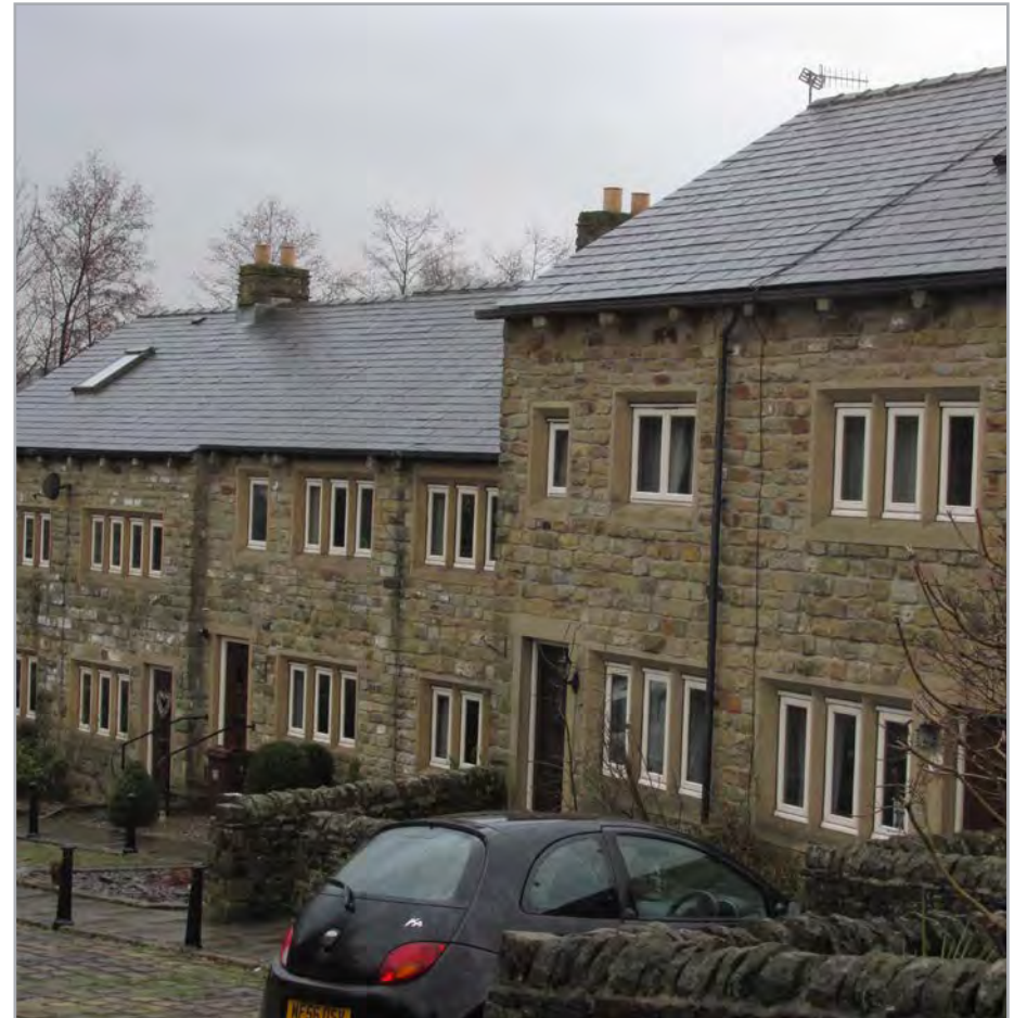
Developed in the 1990s, Bute Street, Old Glossop is a very traditional approach to new development
