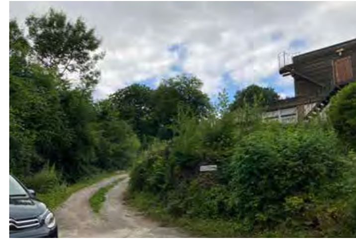
Photograph 11- View of extended gravel driveway and east elevation of the house
